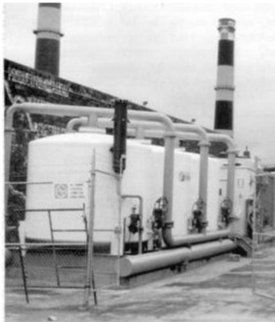
**Figure 4—Three-bed oxygen PSA**
