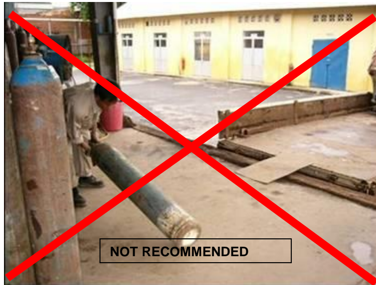
Figure 2 - Bringing a cylinder to vertical position
