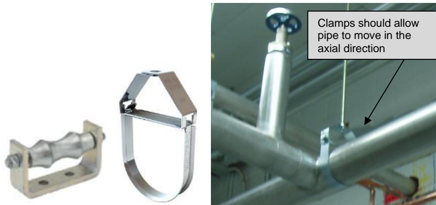
Figure 10 Examples of hangar and roller supports
