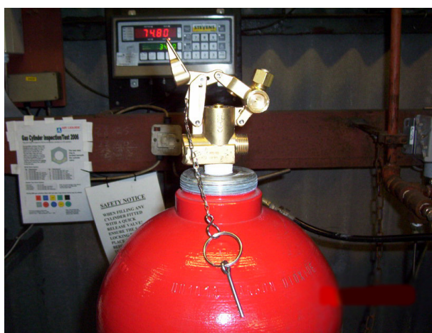
Figure 2—Cylinder valve with locking device disengaged and valve open
