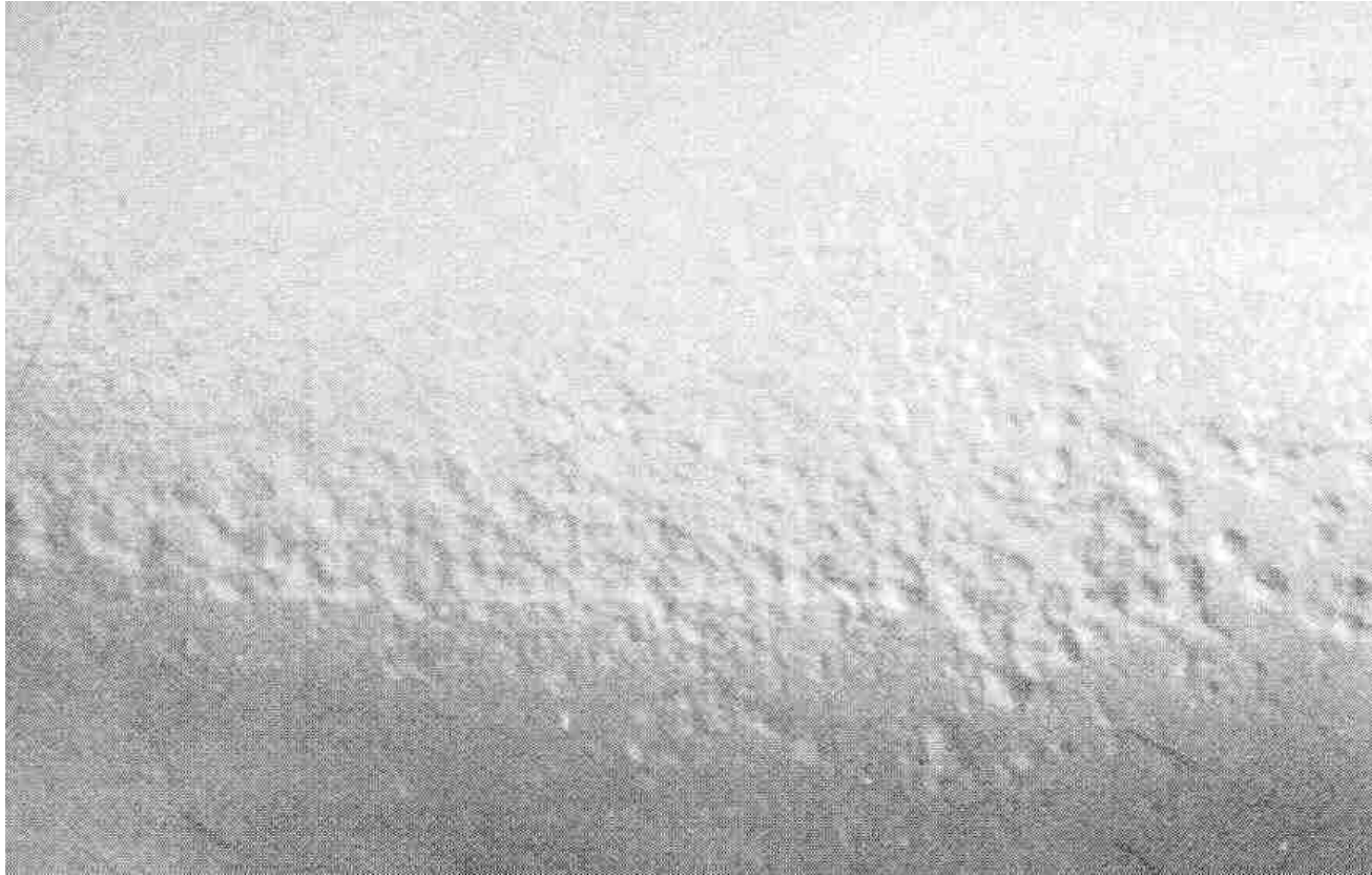
Channel (line) corrosion
