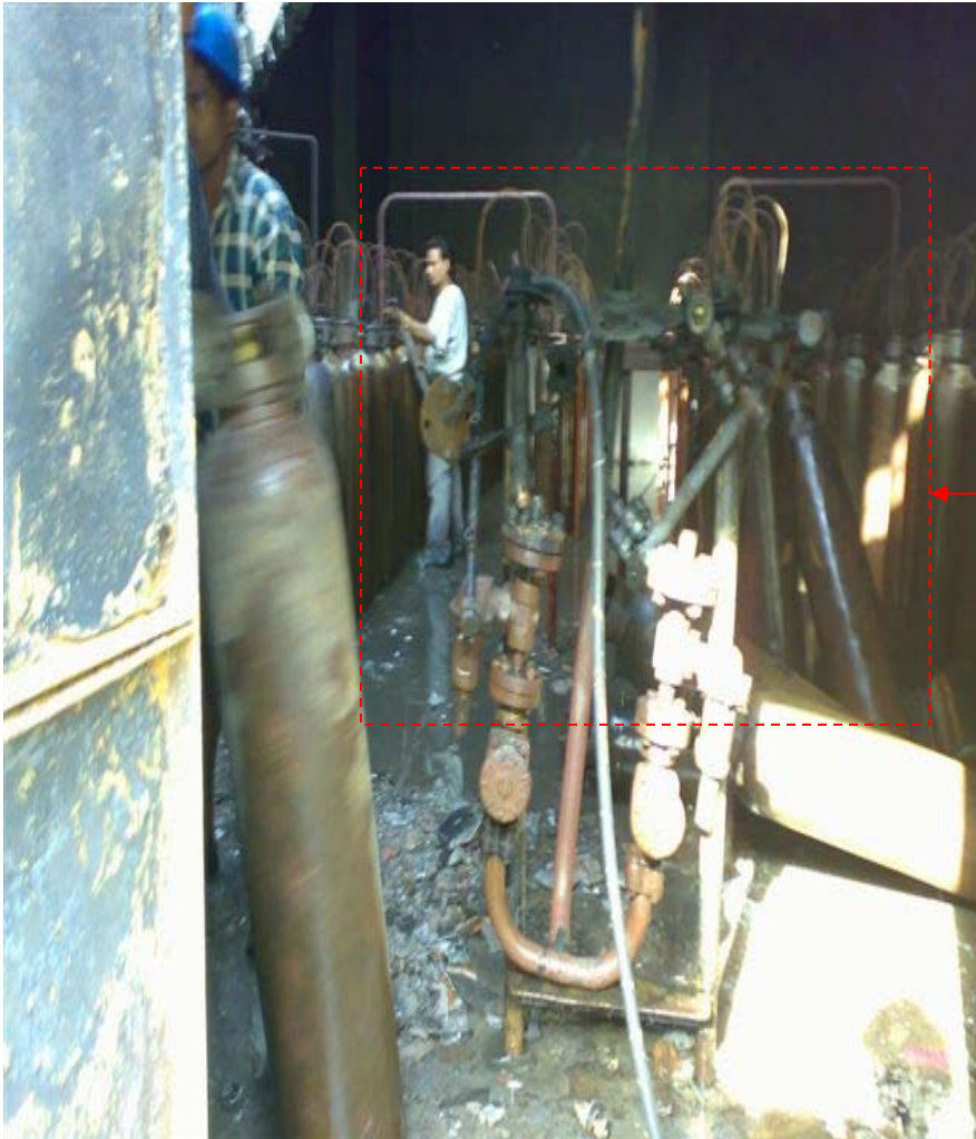
Damaged DA manifold
