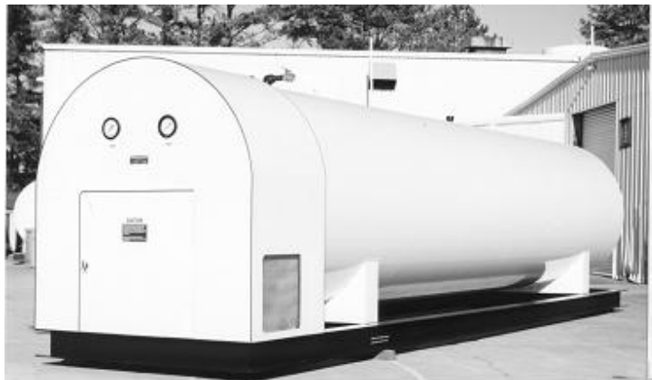
Figure 11—Bulk liquid carbon dioxide container
