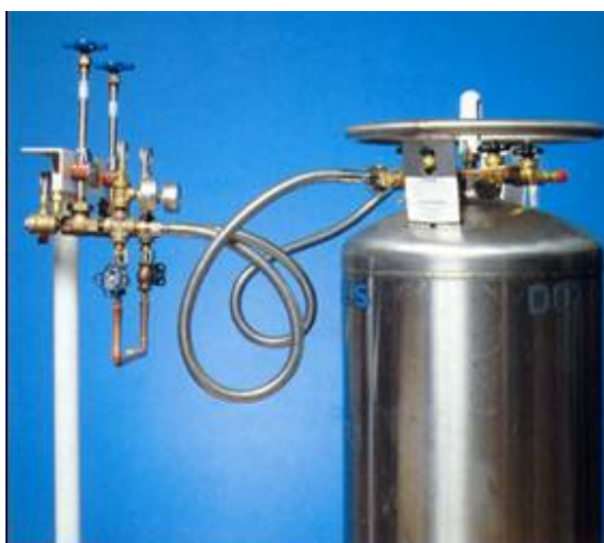
Figure 13—Liquid cylinder fill hose
