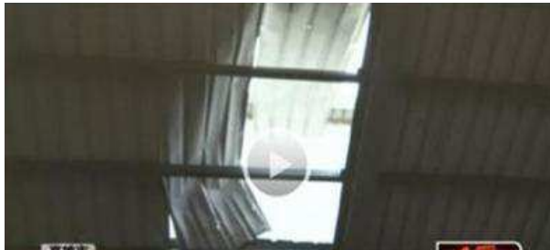
Roof damaged by fragments from ruptured vessel
