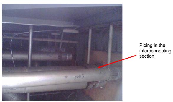
Engineer was found dead in the interconnecting duct between the ASU column and the turbine expander while carrying out a leak check on the piping works and equipment in the enclosure. The plant was undergoing cold test. Engineer was from Operations and was working with the engineering
