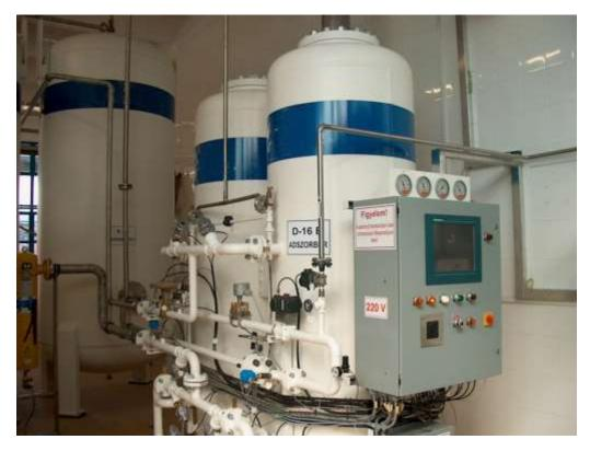
Figure 9—Example of a Nitrogen generator
