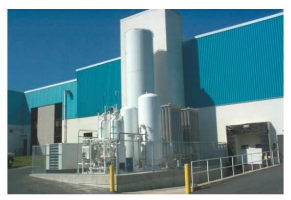
Figure 10—Example of a nitrogen generator (Photo courtesy of Air Products and Chemicals)
