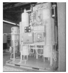
Figure 15—Example of a deoxo system
