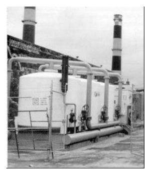
Figure 5—Example of a Three-bed oxygen PSA
