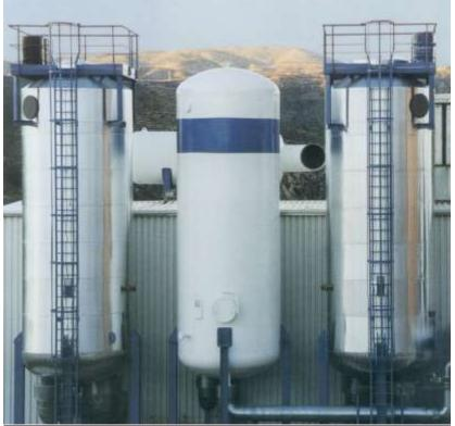
Figure 4—Example of an oxygen VSA
