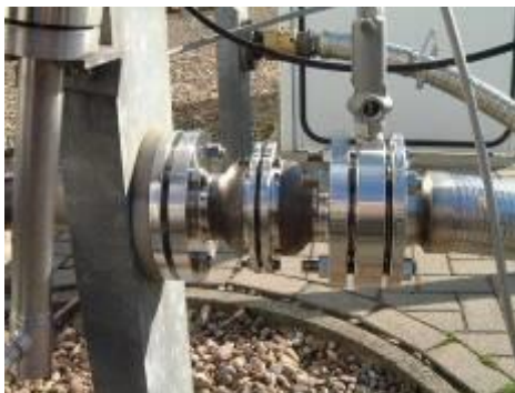
Figure 1 Typical breakaway coupling for liquid filling
