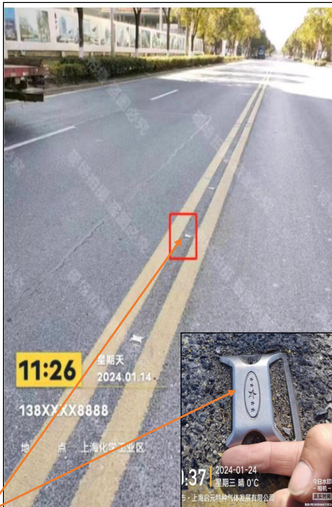
Raised reflective block
