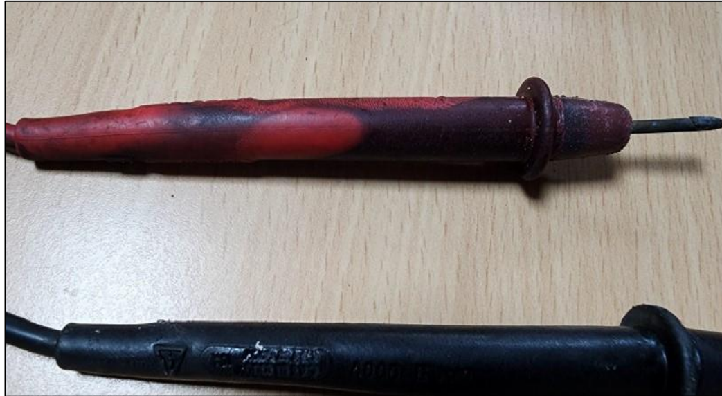
Burnt mark on electrical multimeter
