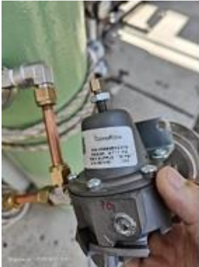
Incorrectly rated pressure regulator
