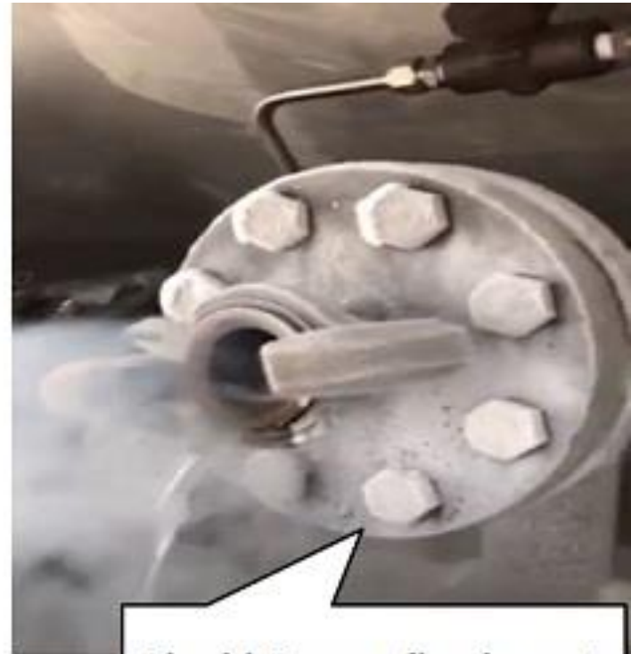
Liquid Oxygen flowing out
