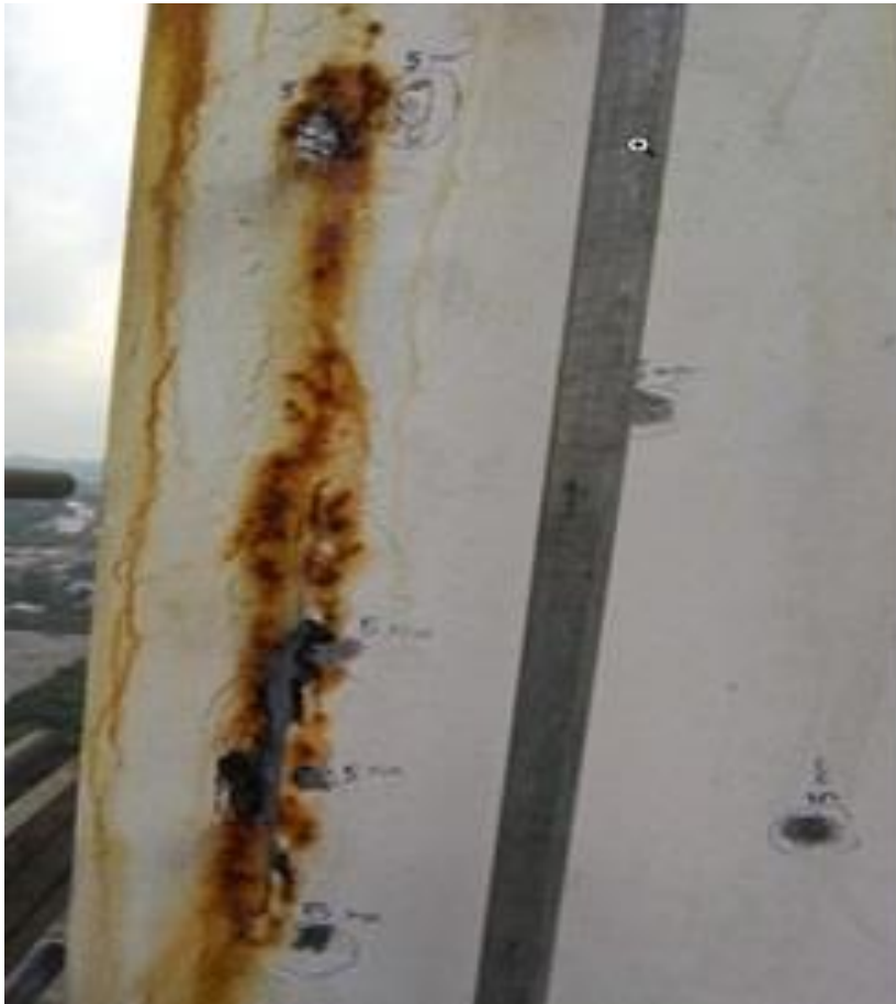
Corroded Casing
