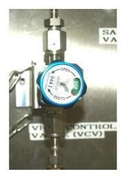
Figure 7 – Manual control valve
