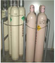
Figure 5 Rack cylinder storage
